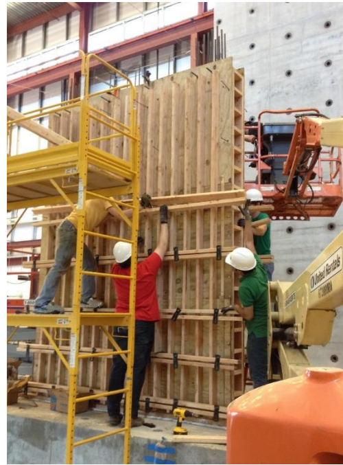
Figure 23 – Lift 1 formwork assembly (T1)
